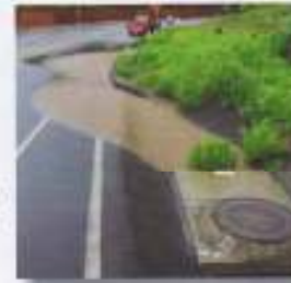
Polluted stormwater runoff flowing into a storm drain.
